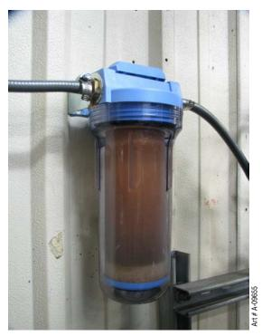
7. Make sure that the hose going to the DMC-3000 is connected to the port on the WMS Water Softener marked "OUT" and the incoming water supply connected to the port marked "IN". Do not mount over any electronics or outlets in case of leaks during operation or spills when changing the element at a later date.
