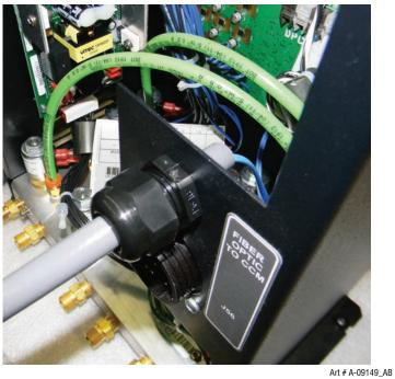
5. Plug the Fiber Optic Cable into the PCB as shown below. Make sure the locking tabs are engaged.
